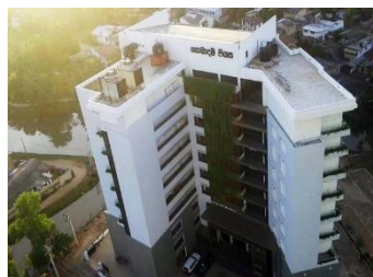
Figure 4.2.4: Front views of the NES building.
