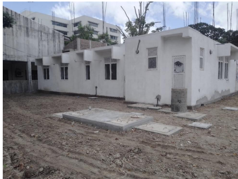
Figure 3- A constructed project with Septic Tank.
