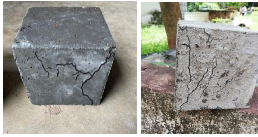
Figure 2: Observed failure patterns of rubberized concrete samples.
