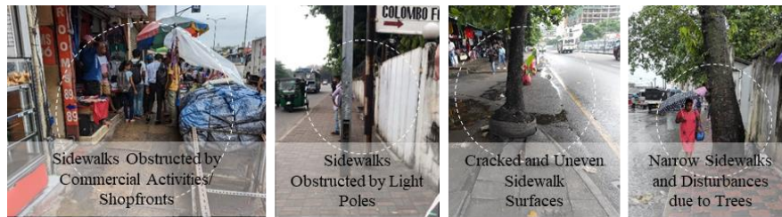
Figure 7: Existing Sidewalk Conditions.
