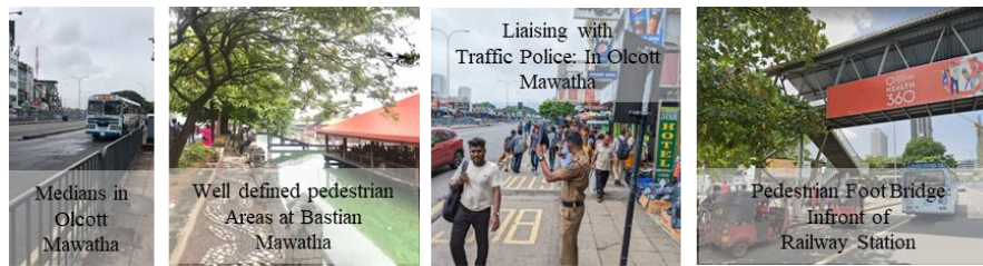
Figure 10: Existing Safety and Traffic Conditions.
