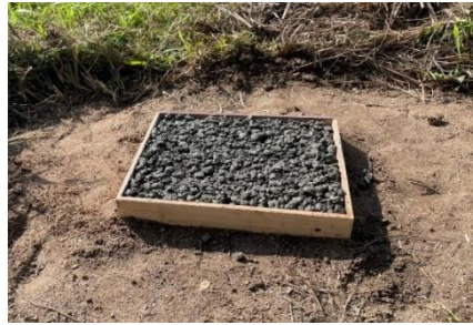
Figure 4: Casted slab panel.
