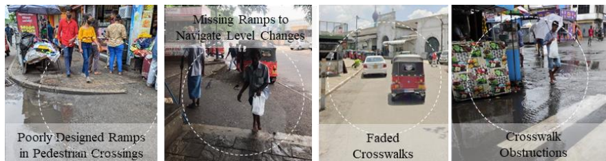
Figure 8: Existing Crosswalk Obstructions.
