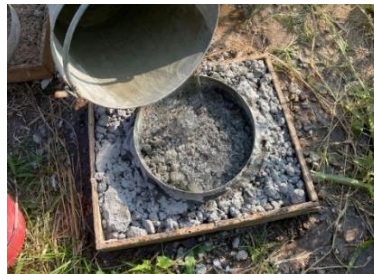
Figure 5: ASTM C1701 Standard Infiltration Test.
