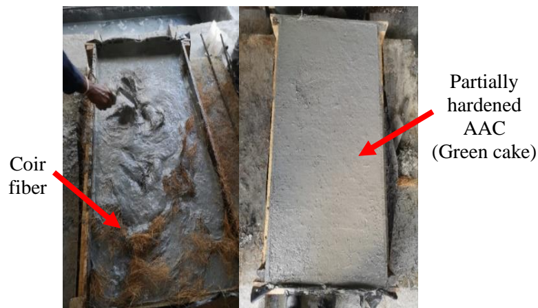
Figure 3.3: Casting coir fiber reinforced AAC wall panels.
